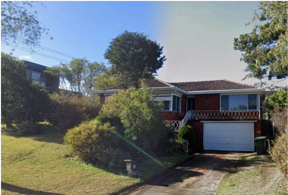
View of existing dwelling at subject site 6 Saric Avenue, Georges Hall
