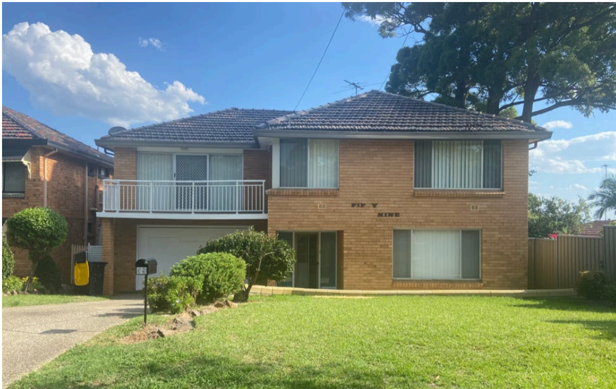
View of rear adjoining neighbouring dwelling at No. 59 Saric Avenue, Georges Hall
